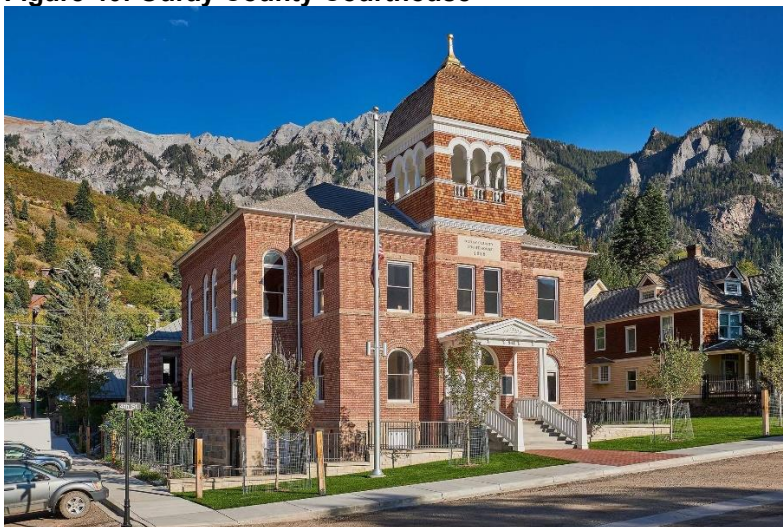
Figure 40: Ouray County Courthouse
