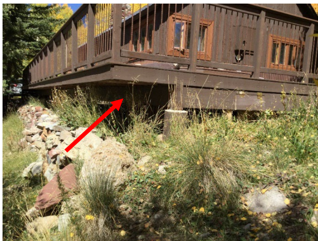
Gaps underneath decks (top left) or decks that overhang (bottom left) are vulnerable to ignition from embers that get trapped below.
