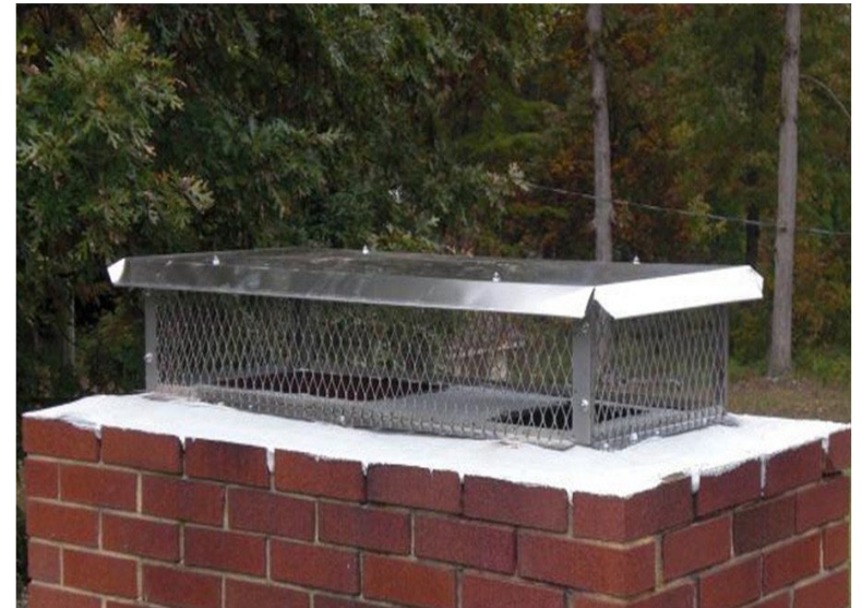
Example of a spark arrester installed on a wood burning chimney to prevent embers from exiting the chimney and to reduce the potential to start an ignition outside of the home.
